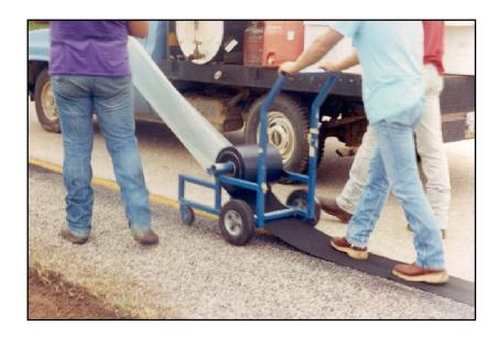
**Polyguard** offers a cart customized to assist in rapid installation of our highway and bridge deck membranes. These carts are adjustable for sizes from 12" – 48" width and are available for purchase and custom made to order.
