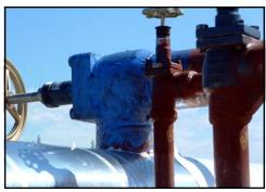
**RG-2400 LT** is not "new" technology, it is new to the insulation industry and a breakthrough for corrosion control and prevention on piping systems, tanks and vessels under insulation. It is a non-drying compound easily brush/spray applied to pipes, fittings, valves, tanks and vessels. It's non-skinning and non-sag properties make it a permanent solution.
