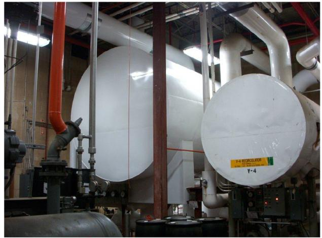
Indoor tanks to be finished with Metal, PVC or Alumaguard Lite. Outdoor tanks and vessels to be finished with Metal or Alumaguard jacketing.
